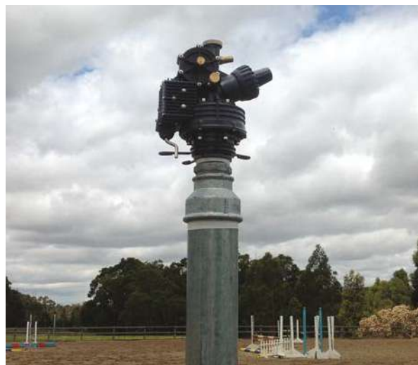
Turbina ST-1600-HS-BR instalada
